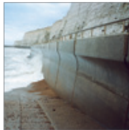
Seawall Brighton (UK), 1992
