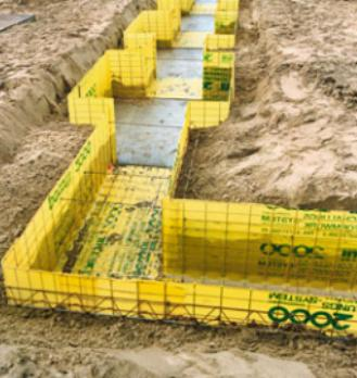
Circular formwork for foundations
