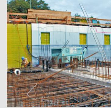
Pecafil partition formwork, optionally with thermal insulation lining
