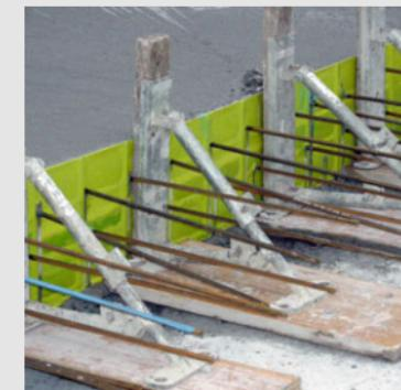
Formwork stop-end with continuity reinforcement
